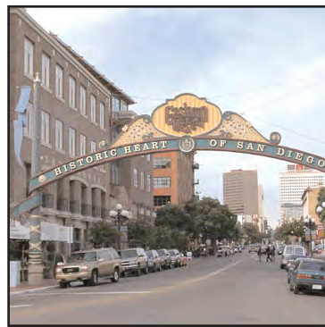
Gateways can consist of signage that extends across streets at key entries to the city center.
